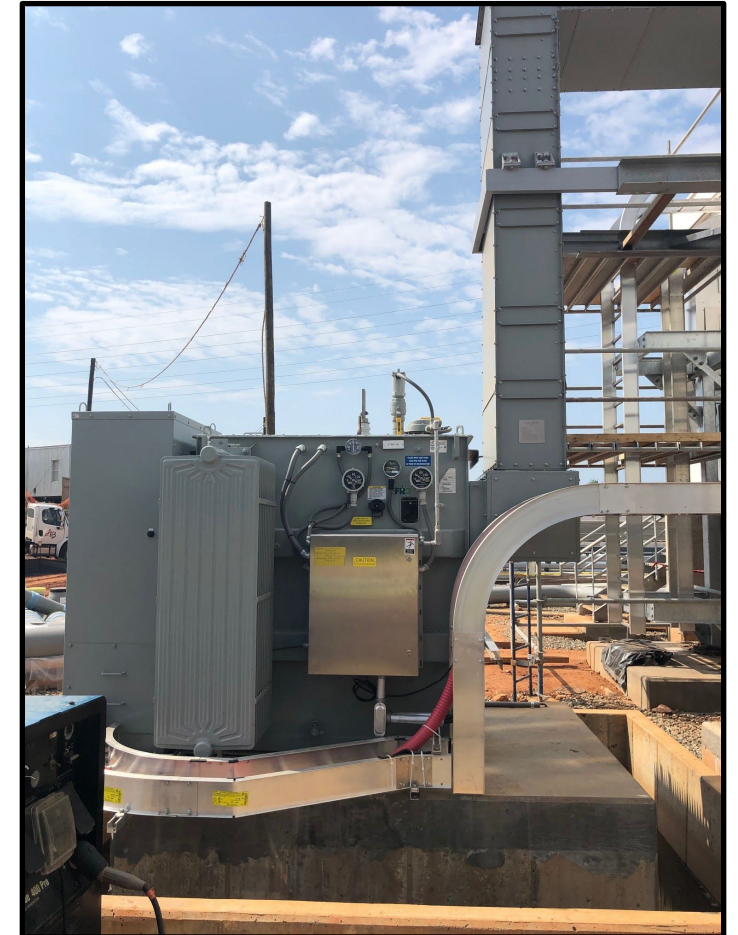
Photos courtesy of Chris Faucette, CMP-17
