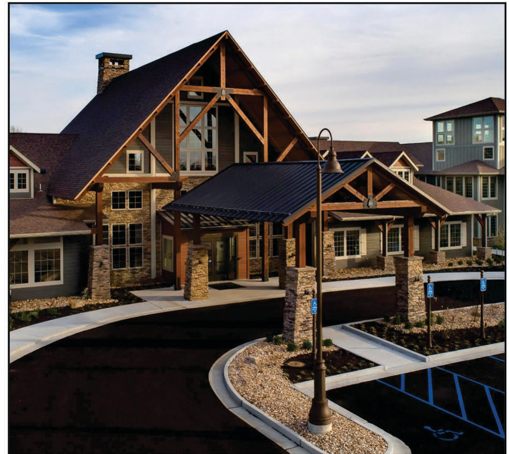
Assisted Living Center (added in 2023 NEC)
