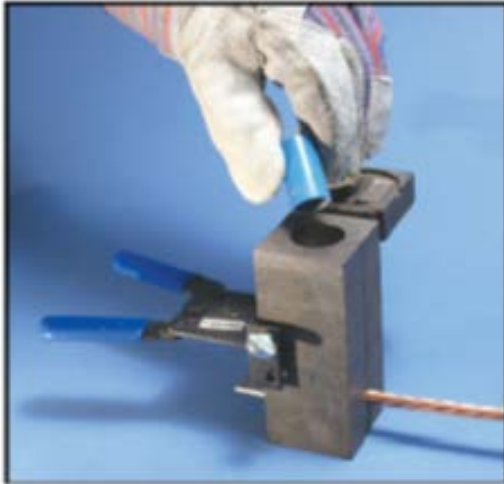
Pouring Weld metal powder into a mold
